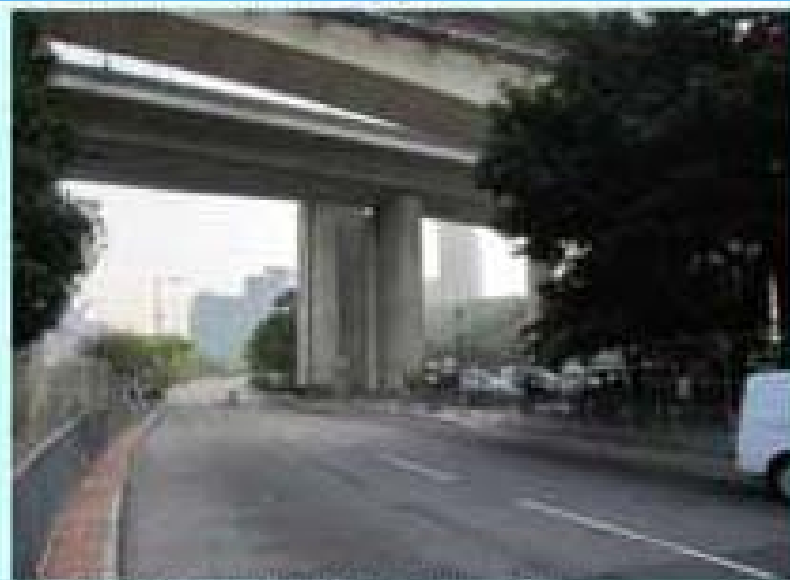
Photo 6: Beneath of Kwai Tsing Bridge.
