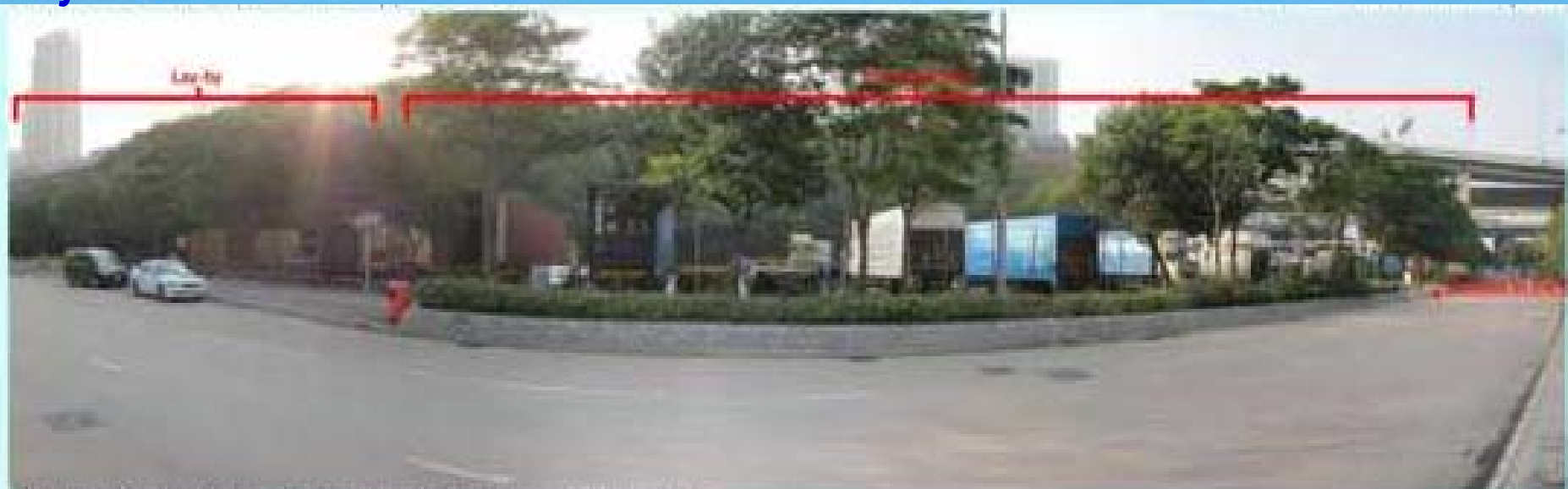
Photo 5: View of the application site from the eastern side.
