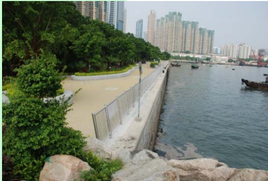
Greening works along typhoon shelter north (completed in Feb 2010)
