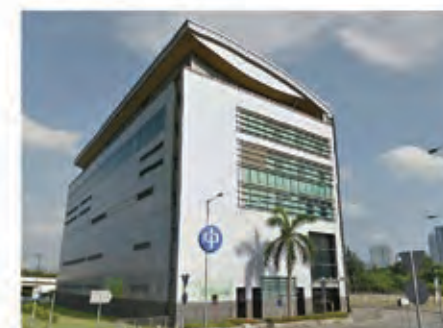
5. CLP CENTENARY SUBSTATION
