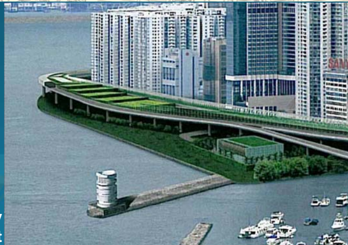
Example of Exhaust Vent Away from Public in North Point
