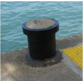
Mooring Bollards (10 tonnes)
