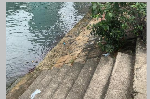
Existing landing steps
