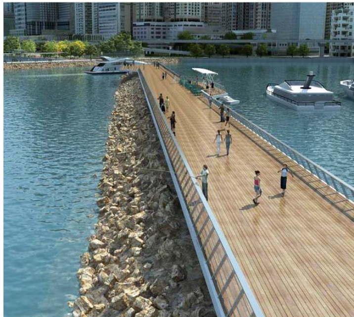
Access to Northern Breakwater
