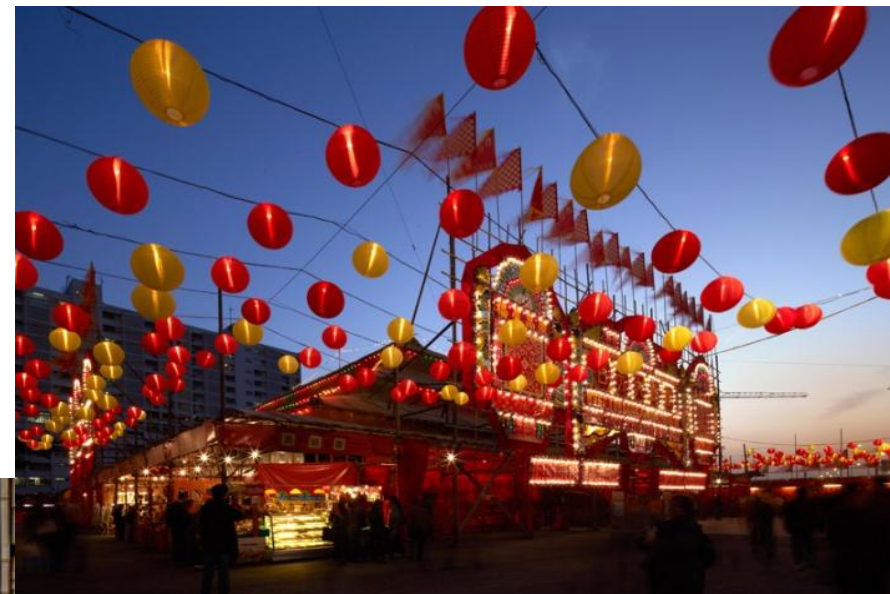
Canopy structures are supported by clusters of bamboo-like metal poles, which allow for festive installations
