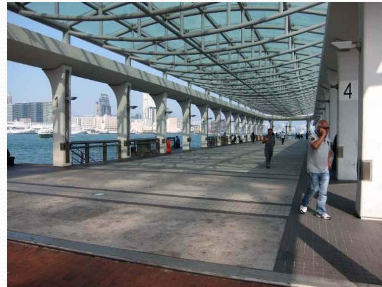
Pier 9 used by the public
