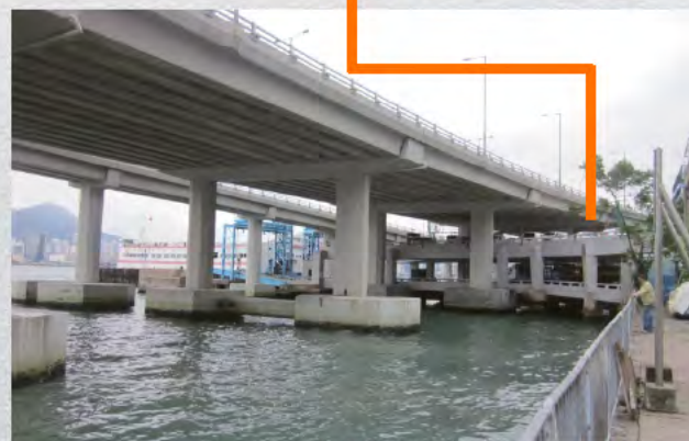
Vehicular Ferry Pier
