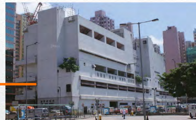
Java Road Municipal Services Building
