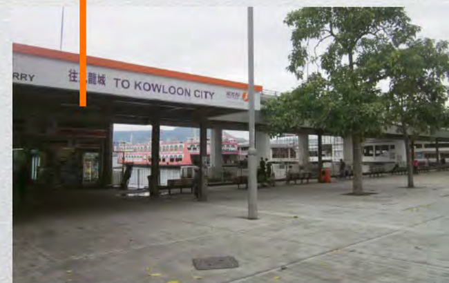
North Point Ferry Pier West
