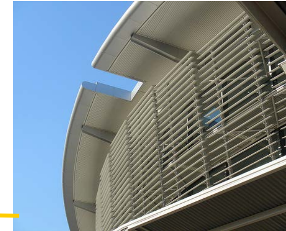
External Louvre Systems - minimise heat gain
