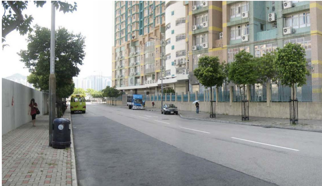
愛德街現狀 Existing (Oi Tak Street)
