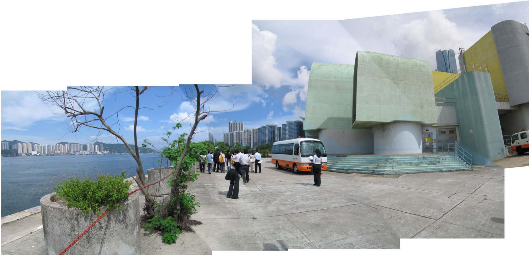
Photo of the Existing EHC Ventilation Building 東隧通風大樓現狀
