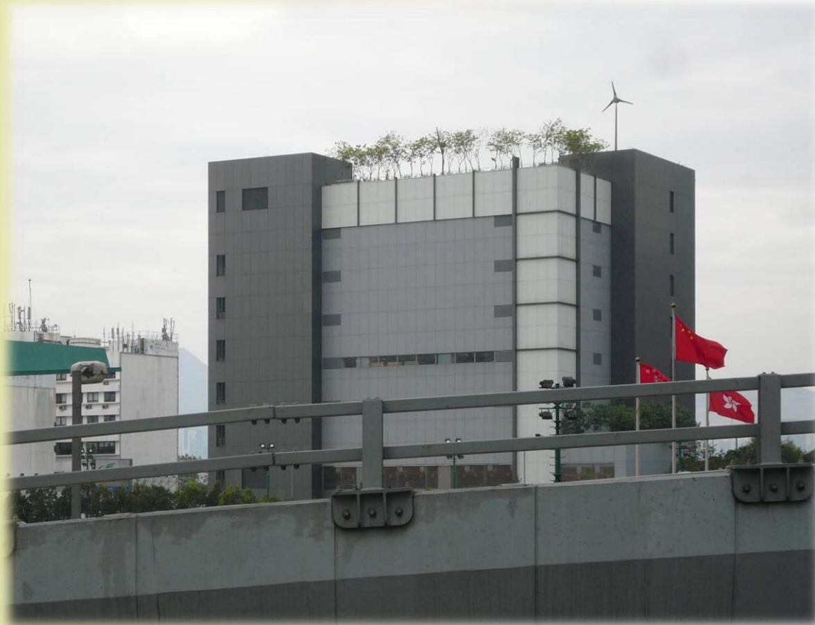
Existing building façade
