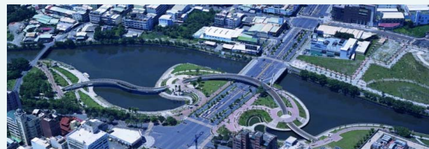
Heart of Love River Footbridges, Kaohsiung, Taiwan
