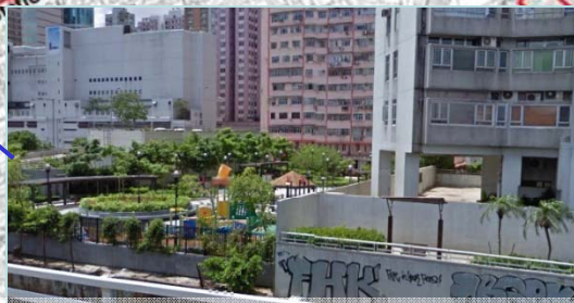
Removing the boundary wall at Provident Centre and Tong Shui Road Garden to connect the waterfront
