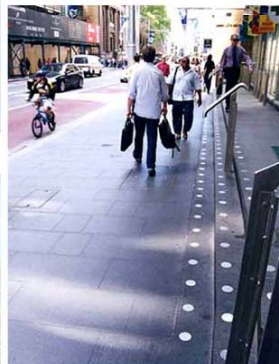
Granite paving and lighting indicating directional and way-finding information
