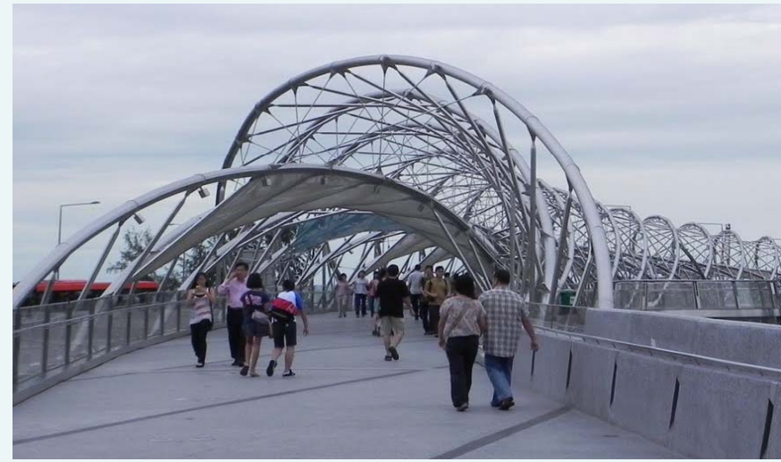
Marina Bay Footbridges, Singapore
