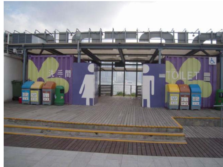
Temporary Washroom 臨時洗手間
