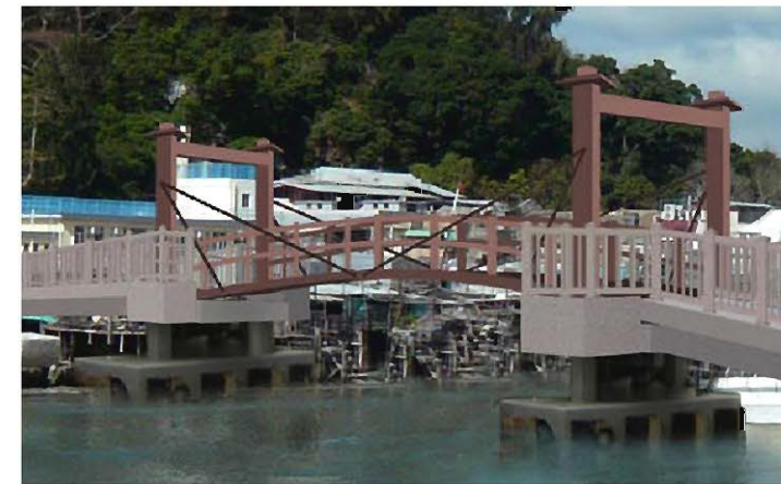
Bascule bridges could be constructed at appropriate locations of the boardwalk to allow access of the vessels to the existing piers adjoining their marine frontage
