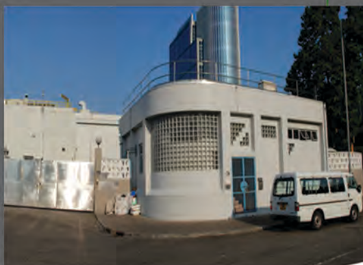
筲箕灣污水處理廠 Shau Kei Wan Preliminary Treatment Works
