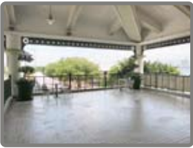
Central Terminal Building 1/F Area: 50.04 m 2
