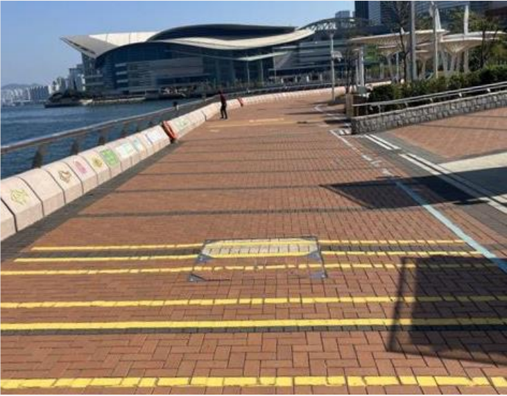
Rumble strip at junction
