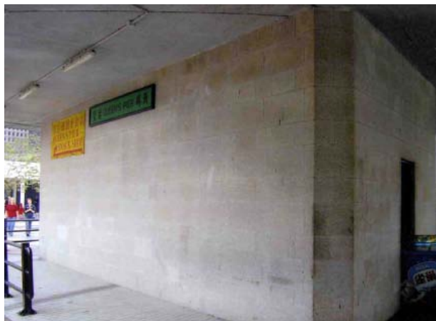
Granite stone cladding on load bearing wall
