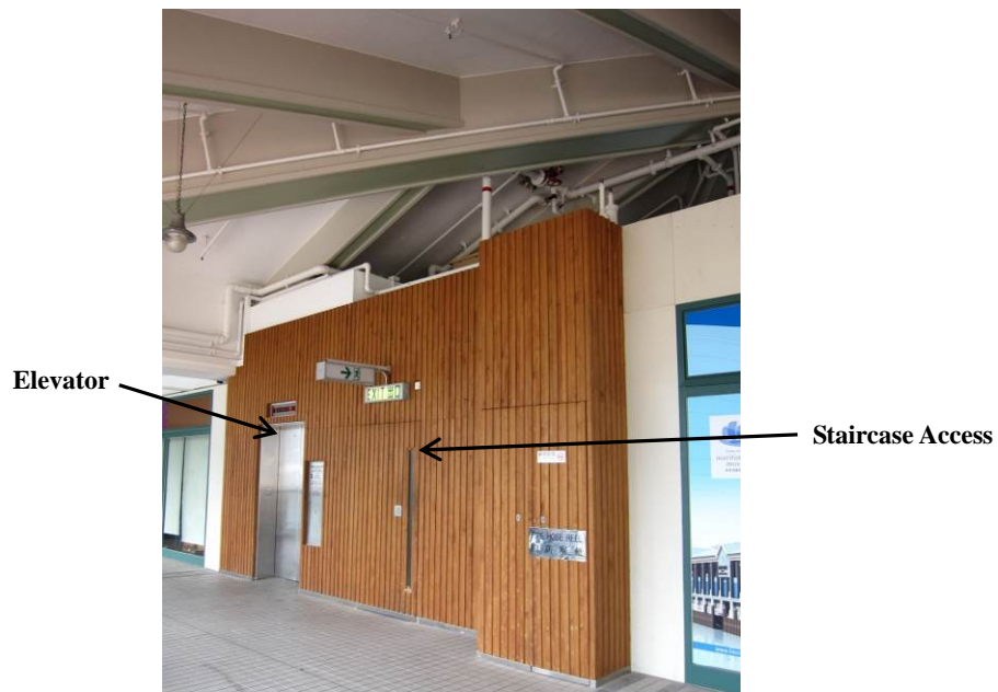
Photo 5: Existing elevator and staircase at the first floor proposed for extension
