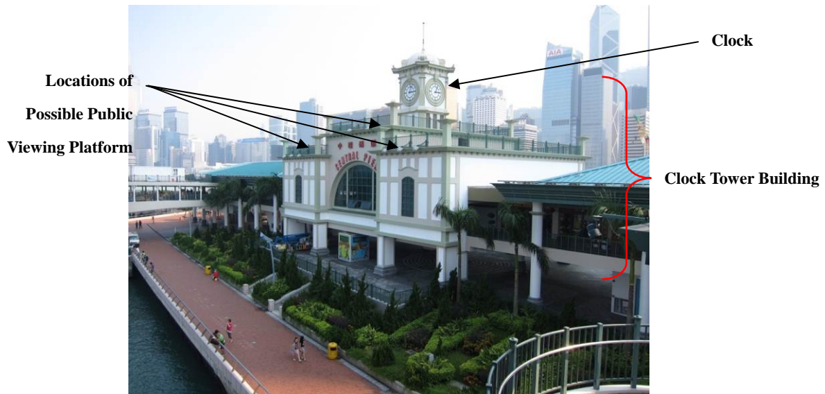
Photo 3: Existing Roof-level of the Clock Tower Building
