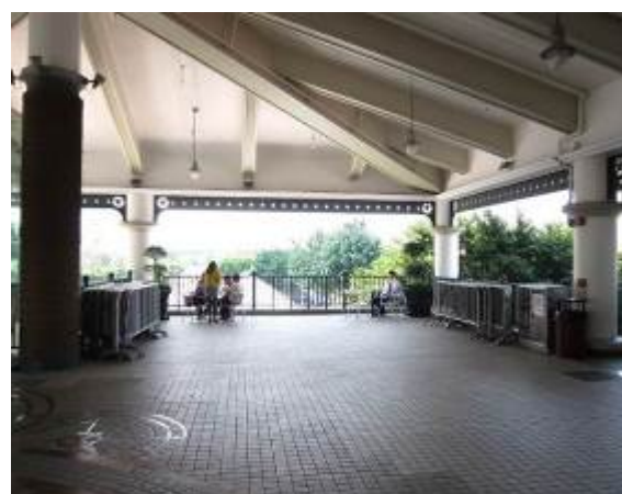
Photo 12: Seating and tables for public use in Central Terminal Building
