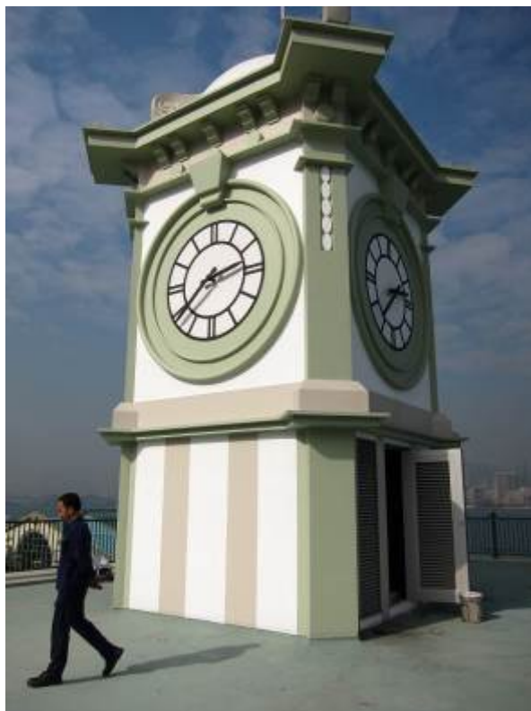
Photo 26: The Clock Tower as an attraction
