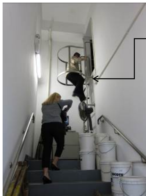
Photo 10: Existing staircase and ladder to roof for maintenance of Clock Tower
