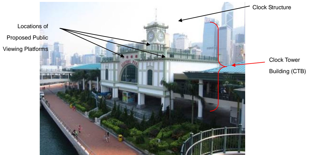
Photo 7: Existing Roof of the Clock Tower Building to which the public currently has no access
