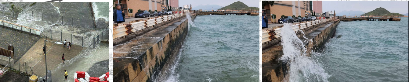
Level about +4.0mPD wave overtopping
