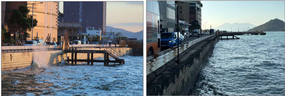
Existing sea wall (about 100+ years) and pier
