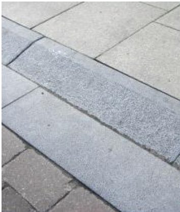
Splayed kerb along footpath
