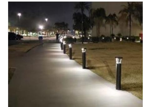
Bollard & Flood light
