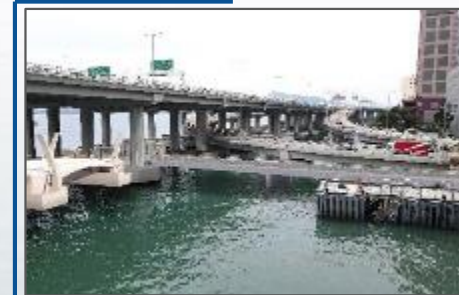
Link Bridge No.2
