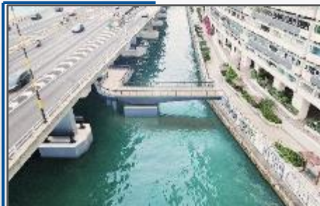
Link Bridge No.1 (Movable - Swing Bridge)
