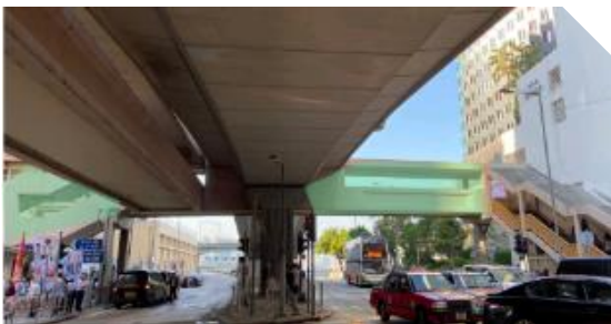
4a. Exterior façade of footbridge
