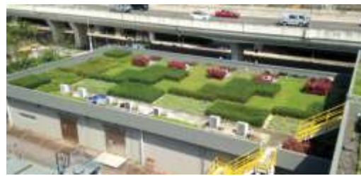
Figure 5 - Green roof at Shatin Sewage Treatment Works
