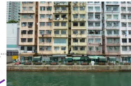
馬頭角海堤附近的私人樓宇 Private buildings adjacent to Ma Tau Kok Seawall
