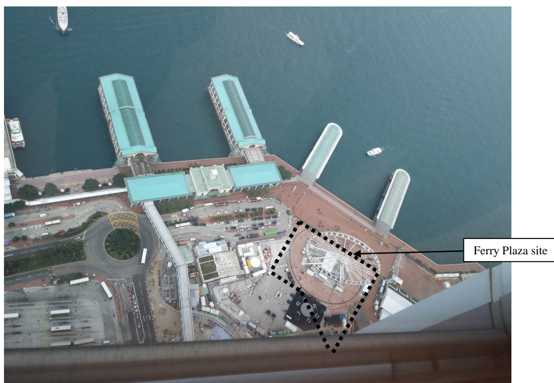
Photo 2: Existing arrangements at Ferry Plaza site (2015)
