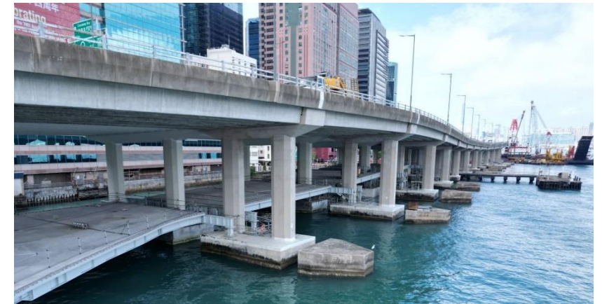
Boardwalk underneath the Island Eastern Corridor (Western Section)
