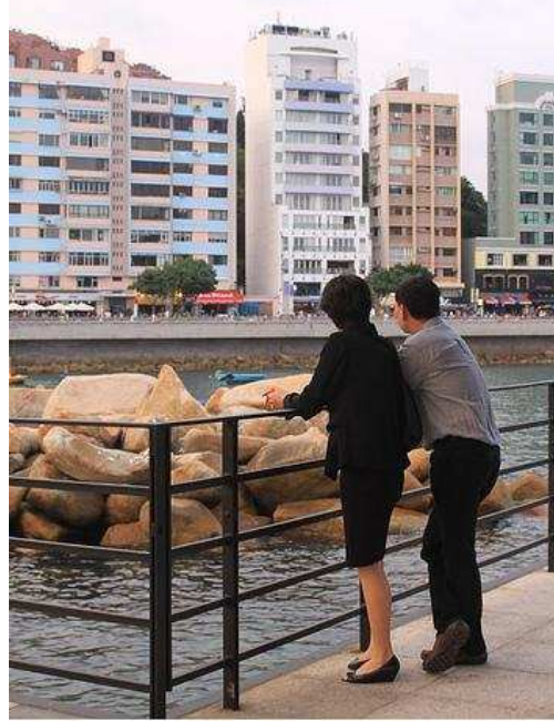
Railing with horizontal infill bars at Stanley, Hong Kong
