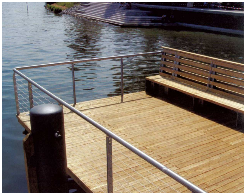
Railing with horizontal infill bars in Potsdam, Germany
